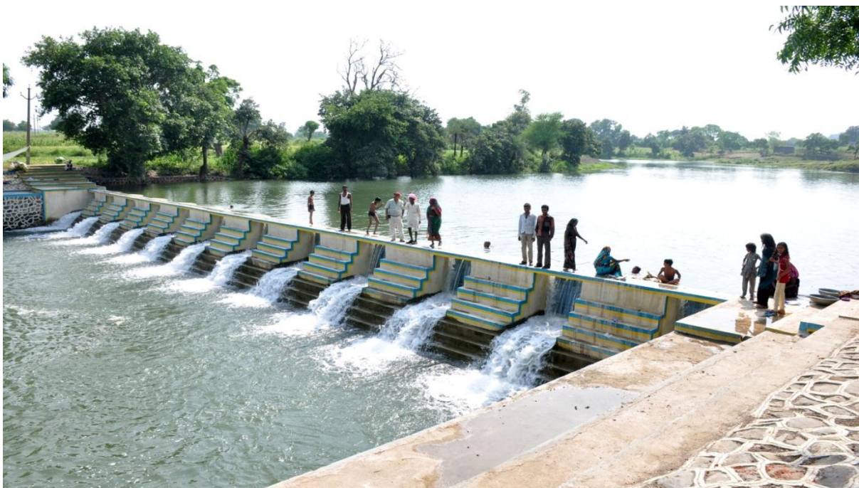
Check Dam – Chhan-II constructed across River Kanthali, in Jhalawar District, Rajasthan.
